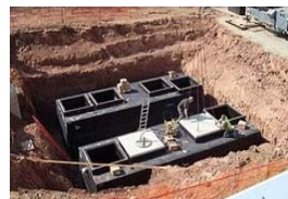
d) Oil and Grease Interceptor - Type 3
