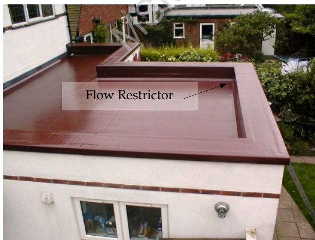
a) Storage Area
