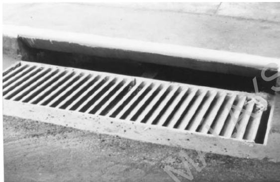
Figure 13.5: Combination Curb-opening, 45 Degree Tilt-bar Grate Inlet
