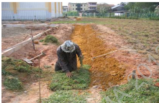
a) Turfing in Progress
