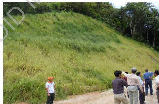
b) Completed Hydroseeding
