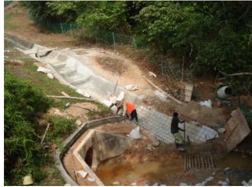
Figure AX2.10: Maintenance Work for Culvert
