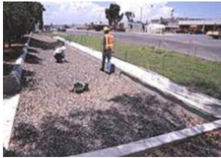
a) Infiltration Trench – Parking lot
