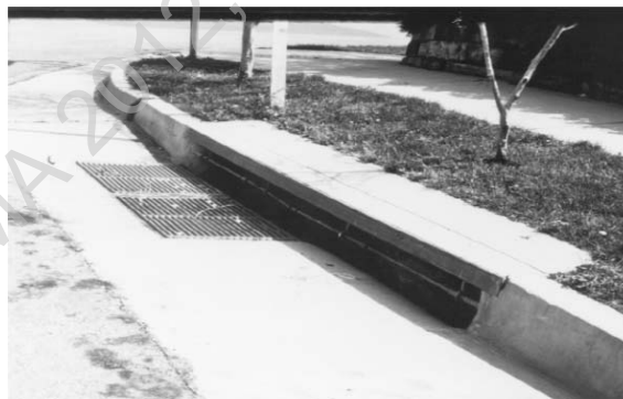
Figure 13.6: Sweeper Combination Inlet
